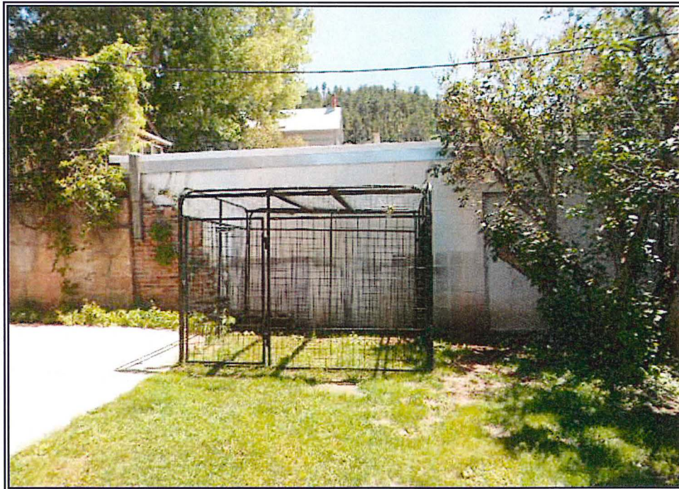
PROPOSED LOCATION OF SHED IN REAR YARD IN LOCATION OF WIRE KENNEL
