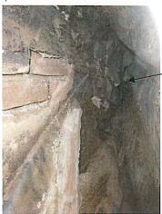
Picture 15 – The membrane had pulled loose from the parapet wall.
