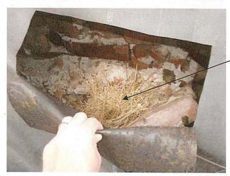
Picture 5 – Northwest corner of roof. Note bird's nest between the membrane and parapet wall.
