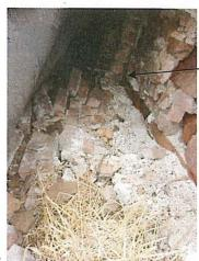
Picture 11 - North parapet wall. Note interior course of brick had fallen away from the wall.
