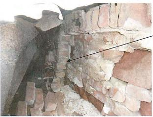
Picture 9 - North parapet wall. Note interior course of brick had fallen away from the wall.
