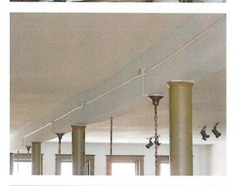
Picture 29 – Note the sag in the roof beam. The sag has occurred over time.
