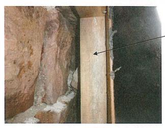
Picture 8 – Wood framing had been added at some point on the south side of the north parapet wall.
