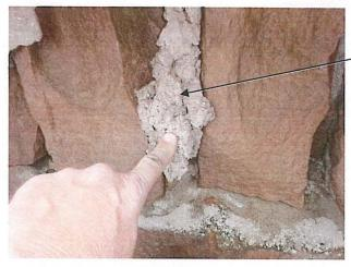
Picture 10 – The original stone parapet wall had been tuckpointed at some point.
