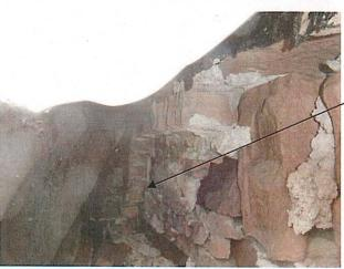
Picture 6 – North parapet wall. Note interior course of brick had fallen away from the wall.
