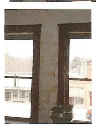
Picture 32 – Water damage was noted between the upper level windows on the north wall.
