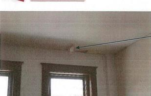
Picture 31 – Water damage was noted on the upper level ceiling at the north end of the building near the northeast corner.
