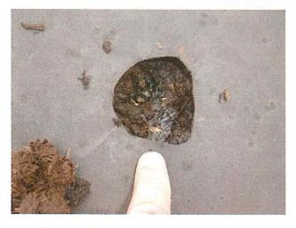
Picture 27 - Roof test core taken near the south end of the building. The fiber board was wet at the test core location.
