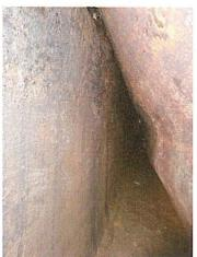
Picture 16 - The membrane had pulled loose from the parapet wall.
