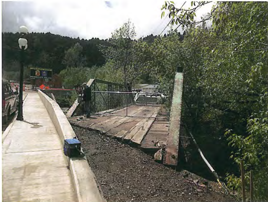
East approach City of Deadwood, Charles Street Bridge 2.JPG 5/25/2016
