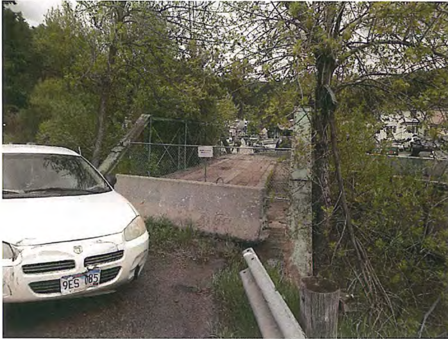
West approach City of Deadwood, Charles Street Bridge 1.JPG 5/25/2016
