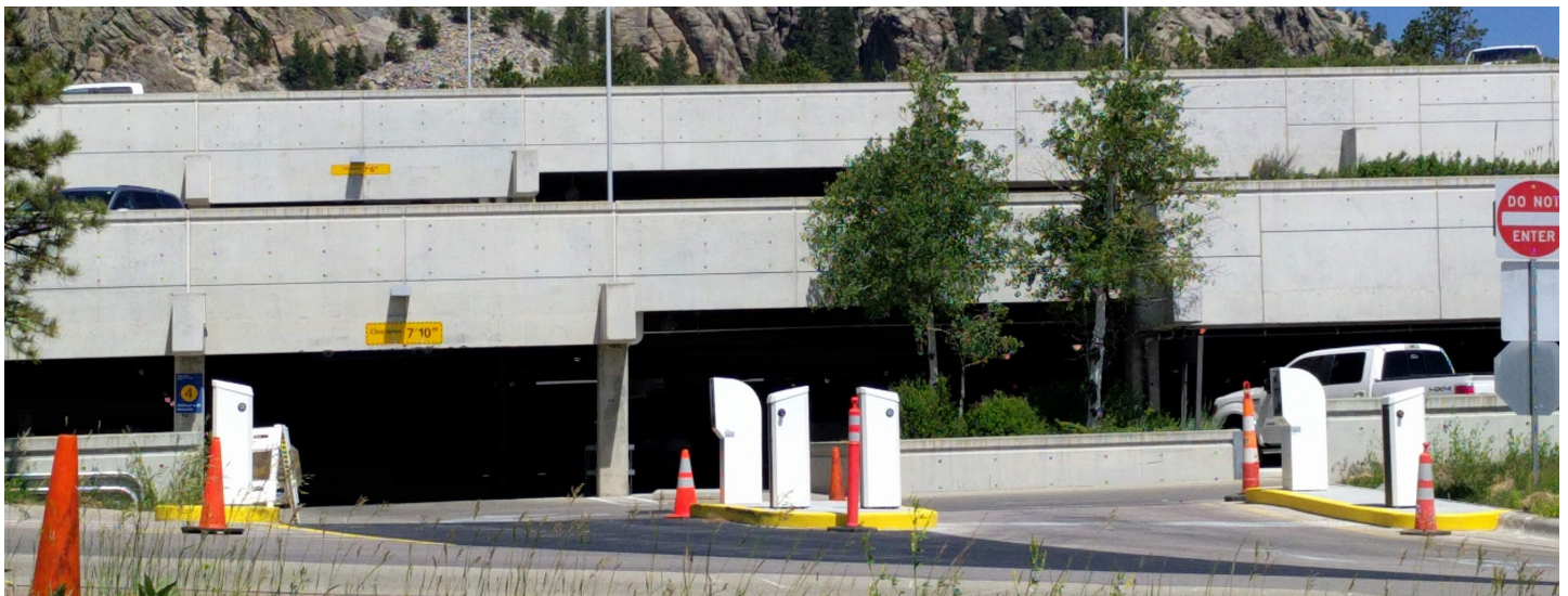
Gated PARCS being installed at Mt. Rushmore ramp.
