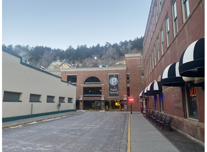
The Broadway Ramp is the largest public parking facility in Deadwood.
