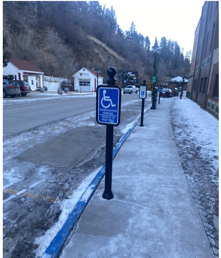
Example of existing on-street ADA spaces. Respondents say there is a need for more ADA parking.
